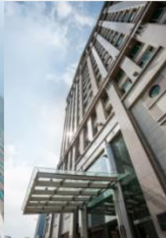
Bugis Junction Towers (100% interest)
