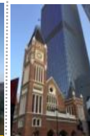
Office Tower on the Old Treasury Building site
