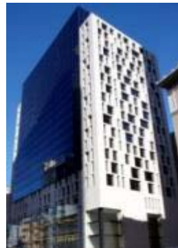
77 King Street Office Tower, Sydney
