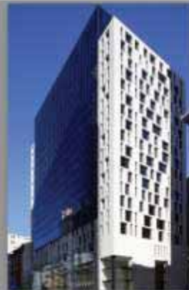
77 King Street Office Tower, Sydney
