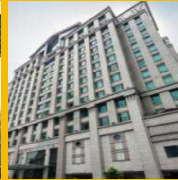
Bugis Junction Towers (100% interest)
