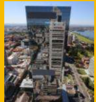
Old Treasury Building Office Tower, Perth (50% interest)
