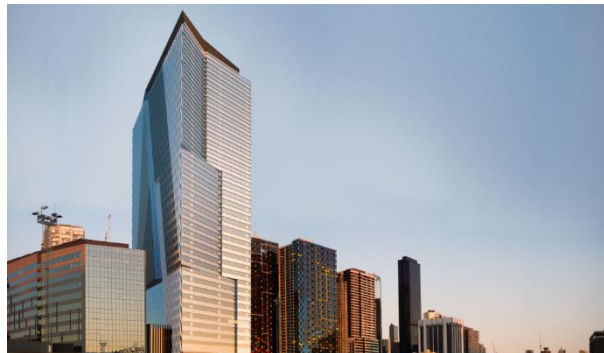
Topped out 311 Spencer Street in Melbourne
