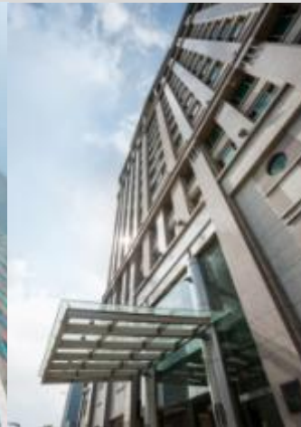
Bugis Junction Towers (100% interest)
