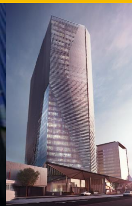
311 Spencer Street, Melbourne (50% interest) -Under construction-
