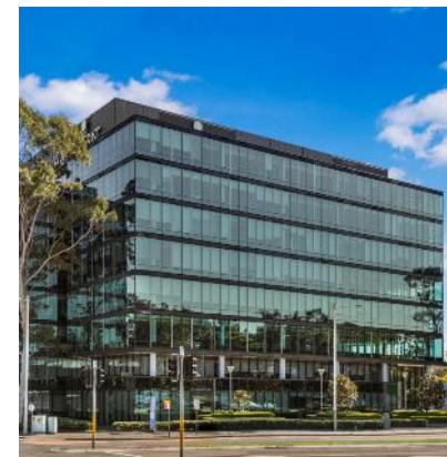
Dec 2020: Acquired Pinnacle Office Park in Sydney
