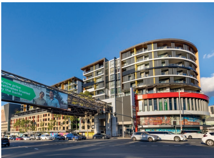
Keppel REIT's first pure-play retail asset, Top Ryde City Shopping Centre, is a freehold suburban mall strategically located in Sydney's City of Ryde.
