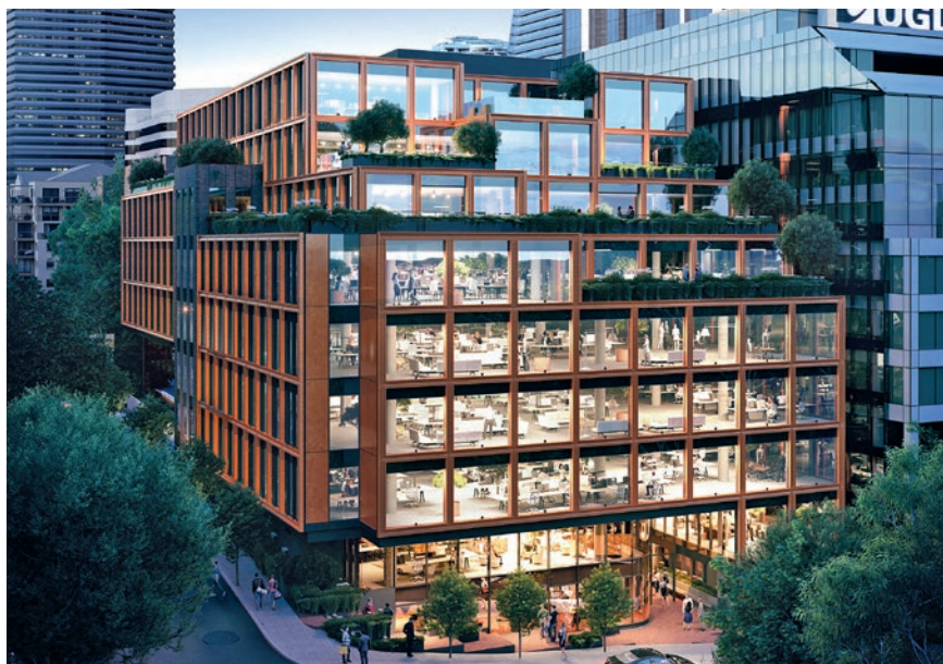
2 Blue Street is a Grade A office building, certified with a 6-star Green Star Design & As Built Rating by the Green Building Council of Australia.
