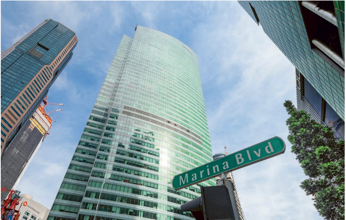
Located in the heart of Singapore's CBD, Ocean Financial Centre is a 43-storey premium Grade A office tower.
